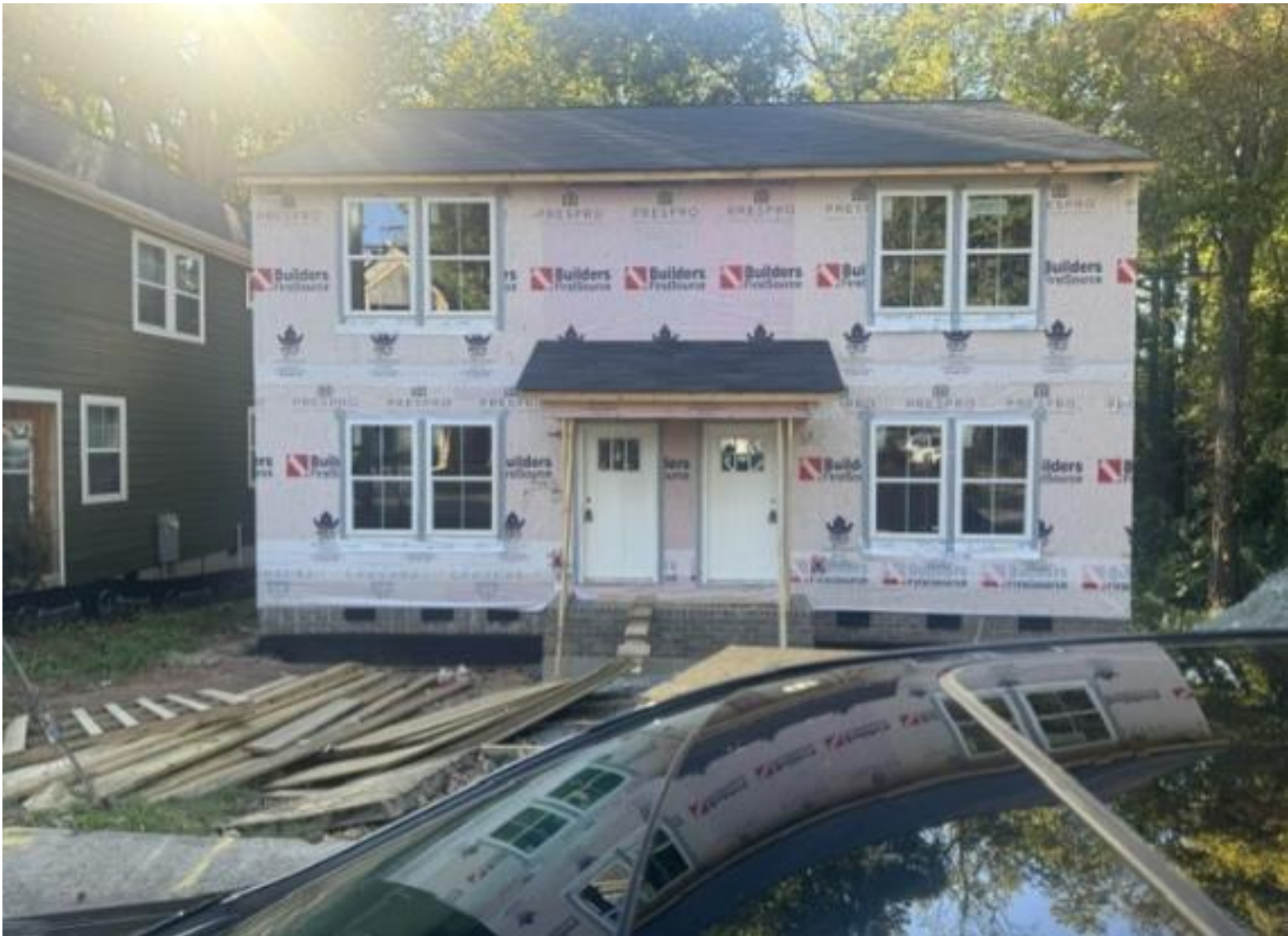
3048 Reid Ave – Duplex unit under construction on previous single family lot.
