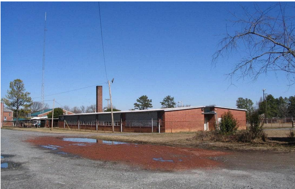
Rear view, 1953 elementary school/cafeteria addition
