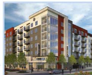
Link Apartments West End Greenville, SC
